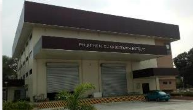
Electron Beam Irradiation Facility
